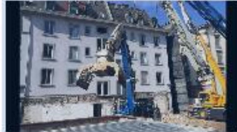
Monitoring under Demolition
